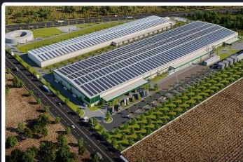
SOLAR CELLS & MODULES PLANT
